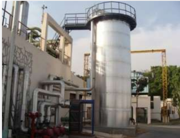
Thermal Energy Storage system
