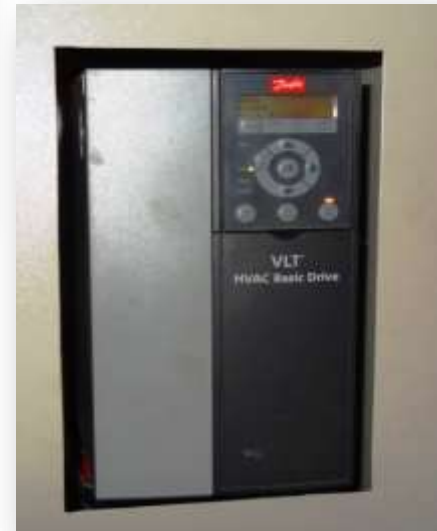
VFD for AHU
